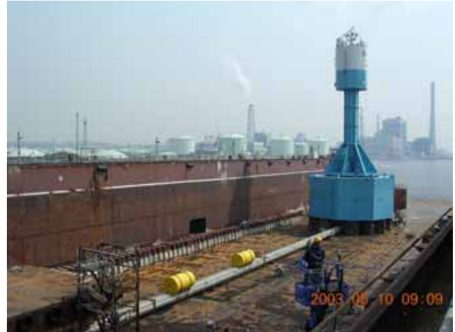
Fig.12 TAKUMI at Final Dock
